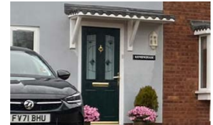
Wood panelled door with small open porch cover.
