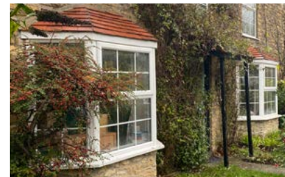
Bay window with red tile capping.
