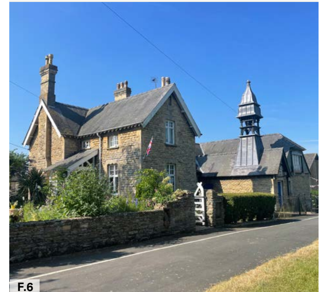
Figure 06: Ingham Primary School's Grade II Listed school house.
