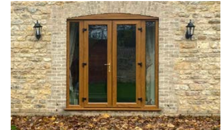
Stable entrance conversion.
