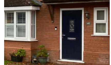
Wood panelled door with open porch cover.
