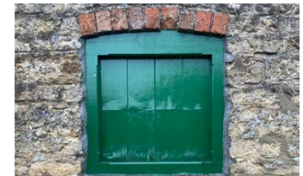
Barn window with red brick decorative arch.
