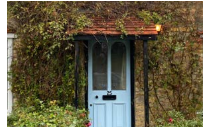
Small open porch with red tile capping.
