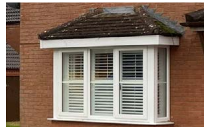
Bow window with tiled capping.
