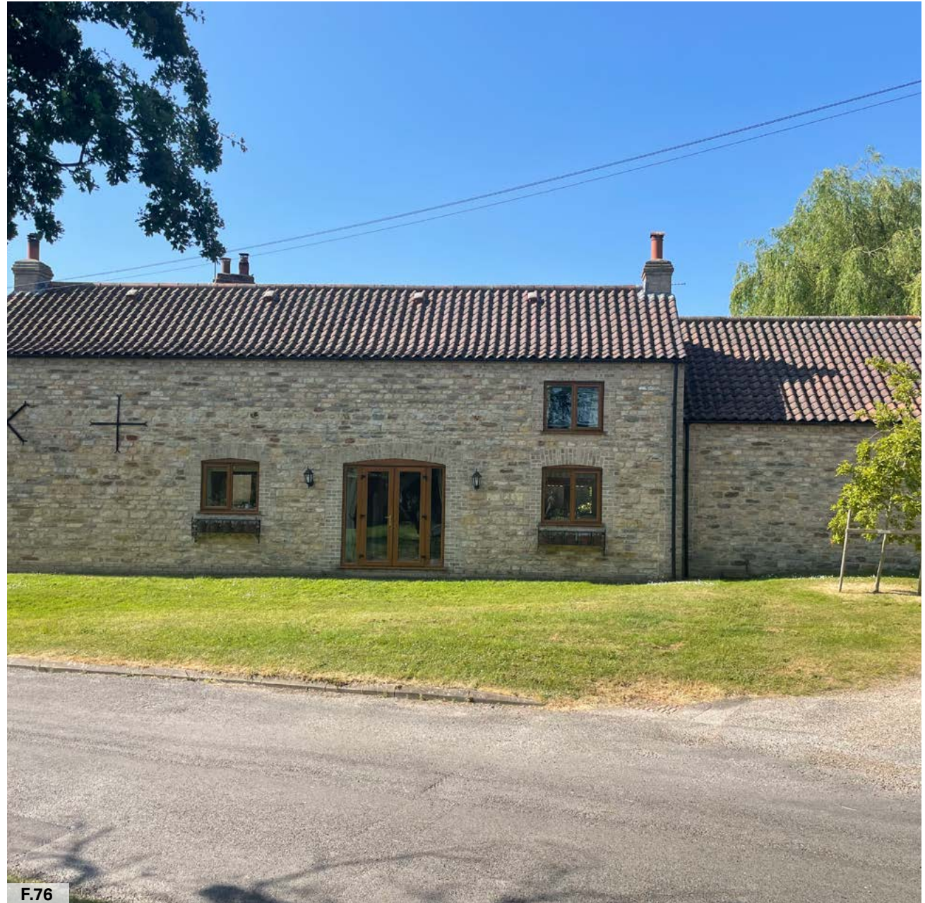
Figure 76: A sensitive barn conversion on West End.
