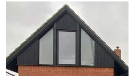
Floor to ceiling modern windows.
