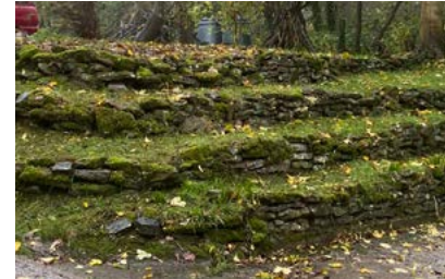
Tiered boundary leading to elevated property.
